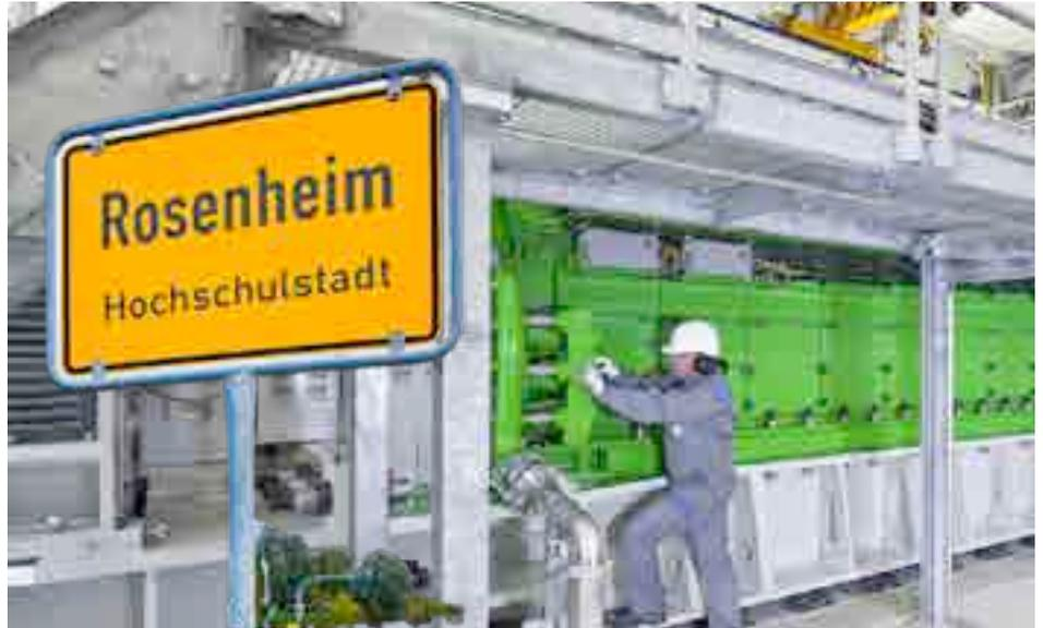
The J920 FleXtra gas engine adds another 9.5 MWel to the Stadtwerke Rosenheim’s installed capacity. Three J620 gas engines (3 x 3.35 MWel) as well as one J624 two-stage turbocharged gas engine (4.4 MWel) were installed in previous years.
