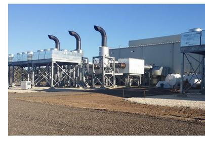
» The Jenbacher technology allows us to quick start the power plant in less than 5 minutes to support grid stability and supply 51 MW to San Bernard's members. This helps provide secure and reliable power to approximately 20,000 homes in the San Bernard region. Plus, the power plant also helps to heat the homes via electrical baseboard or heat pumps.«
