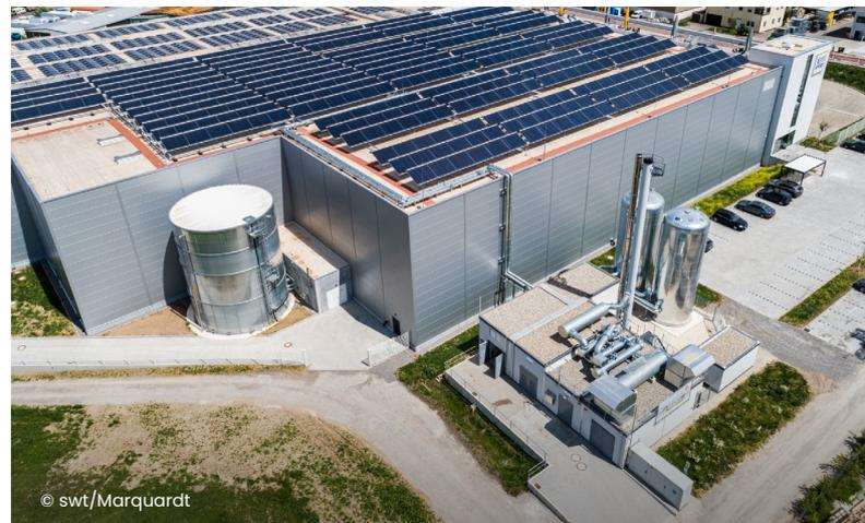
In total, an extra 175 kW of usable thermal output can be heated using the heat pump. The system is enhanced by a 3,000-kW peak load boiler and two large heat accumulators.
